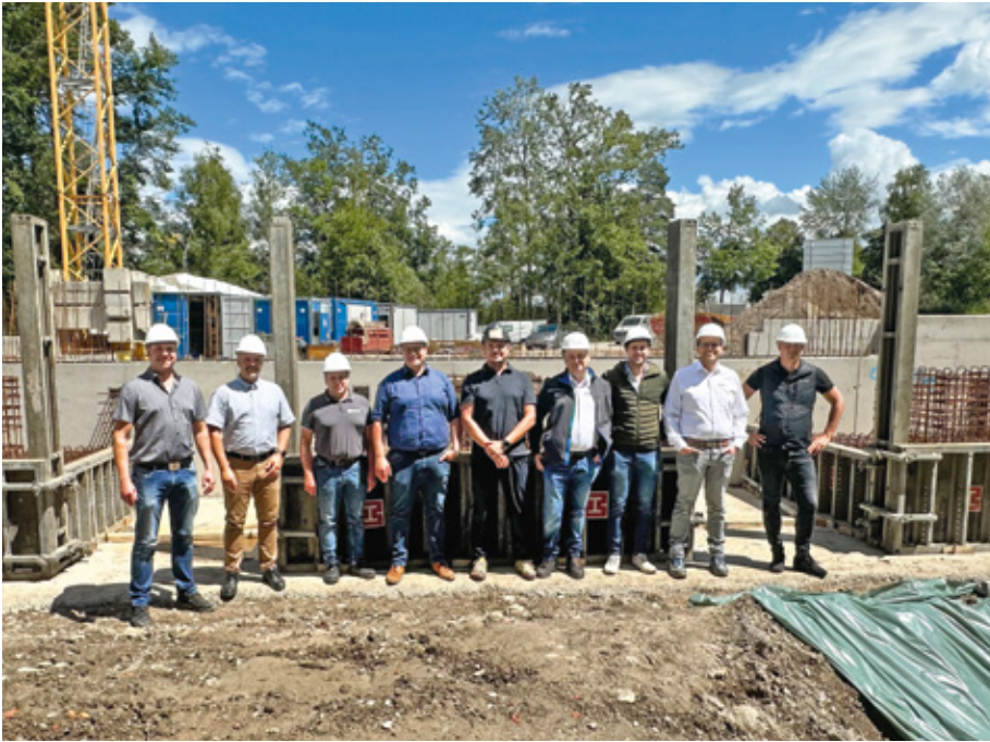
Spatenstich in Bad Feilnbach
